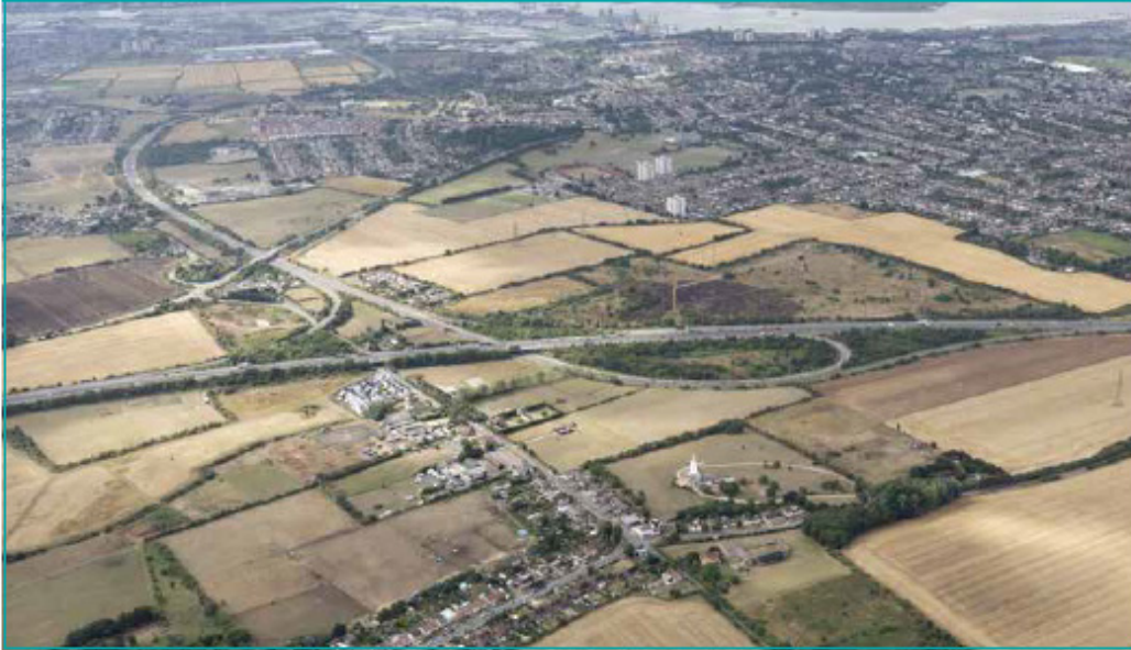
Figure 5-43. Existing A13/A1089 junction, looking south
