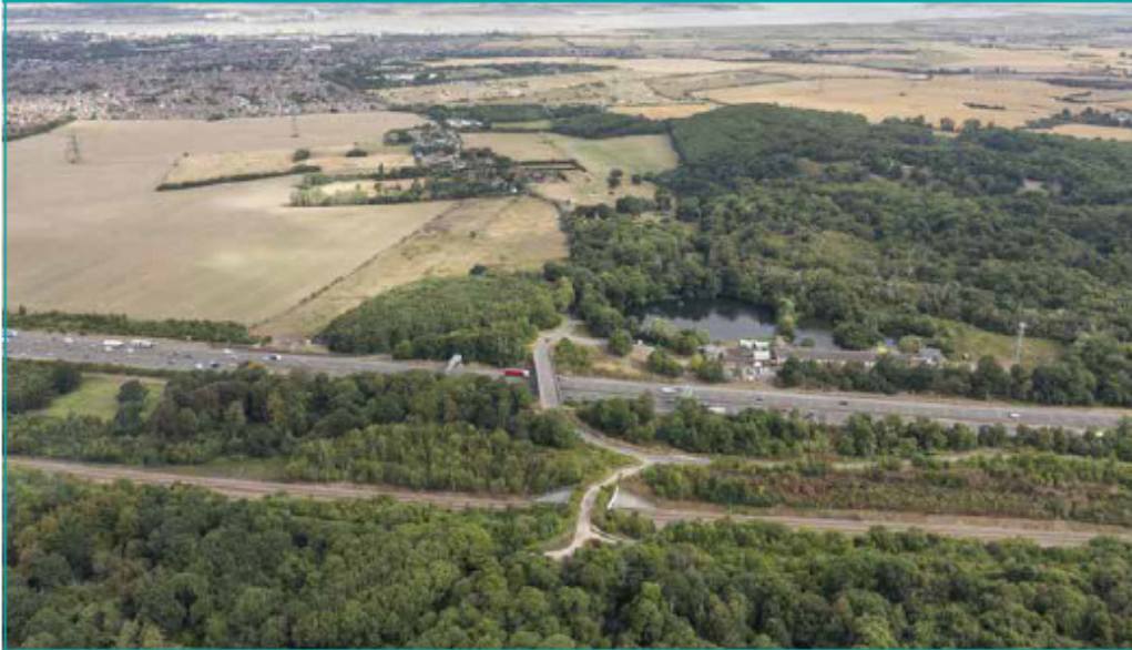
Figure 5-17. Existing Thong Lane and A2, looking north
