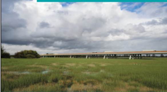
Proposed Mardyke viaduct and wetland creation, from the Mardyke trail, looking north
