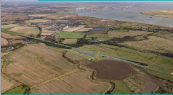
Previously proposed location of Tilbury junction looking north-east from Tilbury Power Station
