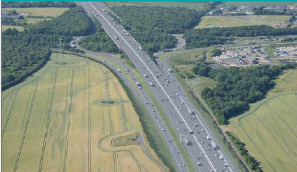
Figure 5-60. Statutory consultation – proposed M25 between junction 29 and 30, looking north
