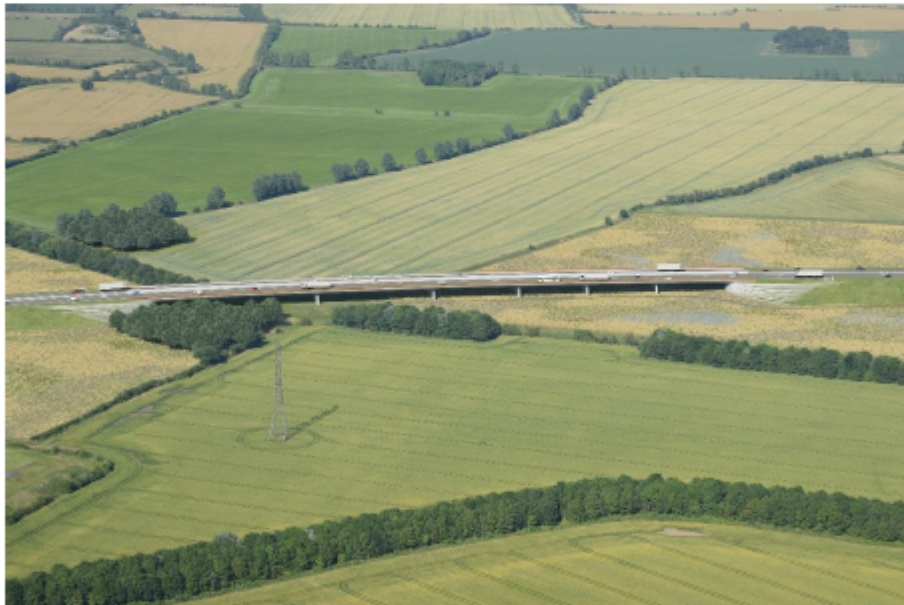
Caption: this viaduct will carry the new Lower Thames Crossing route over the Mardyke valley
