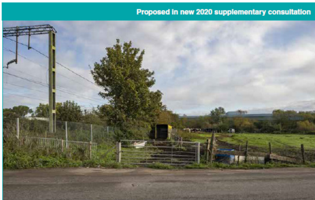
Figure 5-37. Supplementary consultation – proposed Tilbury viaduct from properties on Station Road, looking north-east
