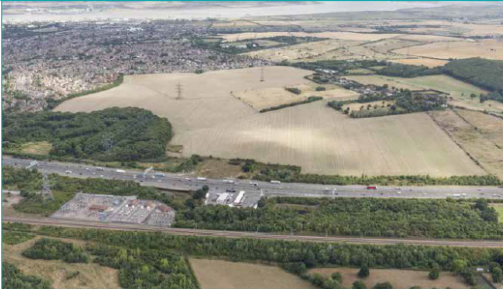
Figure 5-14. Existing A2, looking north
