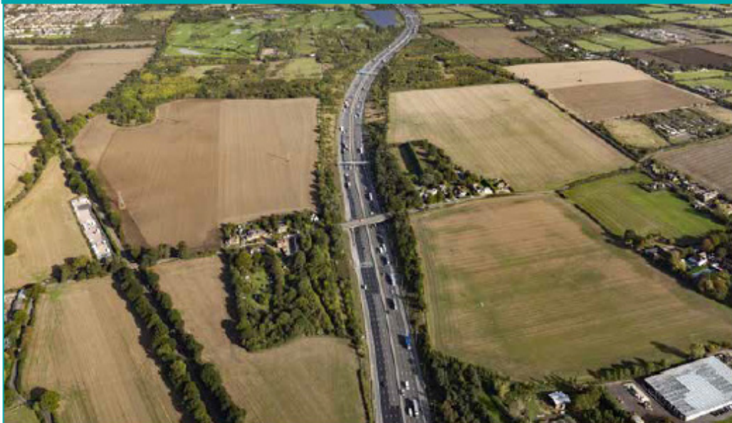
Figure 5-57. Existing M25 and Ockendon Road, looking north
