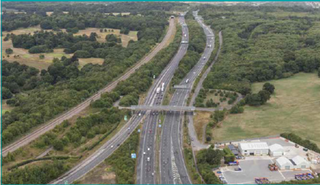
Figure 5-11. Existing M2/A2 along the A2 near Park Pale bridge, looking west
