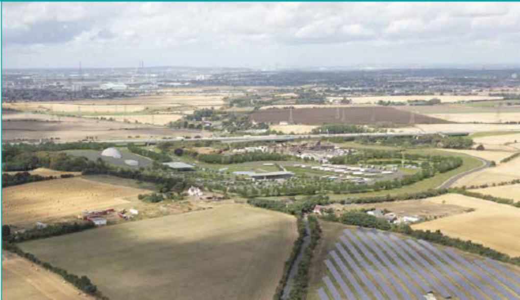
Figure 5-31. Previously proposed Tilbury junction and the rest and service area, looking west
