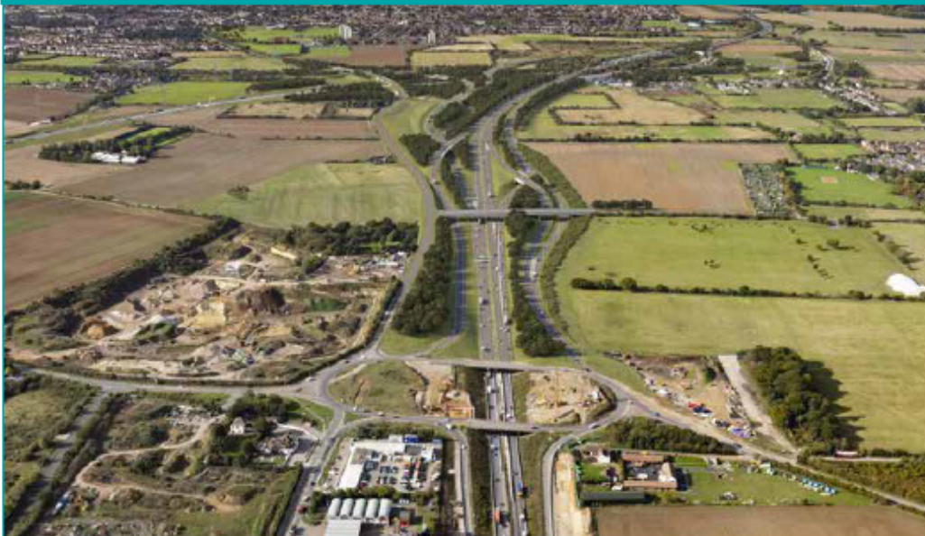
Figure 5-47. Supplementary consultation – proposed A13/A1089 junction at the Orsett Cock roundabout, looking west
