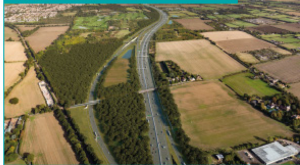
Proposed LTC/M25 junction, with the new Ockendon Road bridge, looking north
